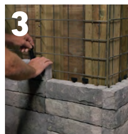
3 Attach Tandem Veneer with Connector
